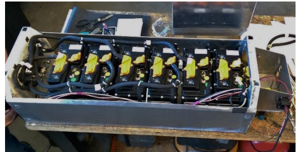
Figure 4: The aluminum battery container houses 6 batteries, and is located on the top of the tunnel.
