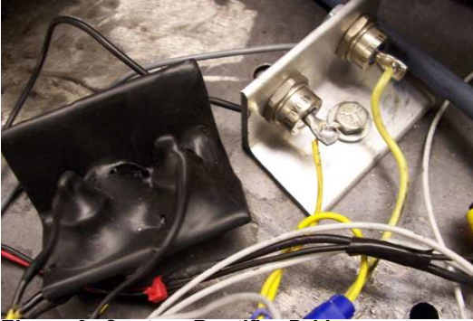
Figure 8: Custom Rectifier Bridge
