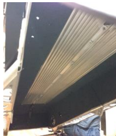
Figure 22: View of tunnel underside lined with Lizard Skin material
