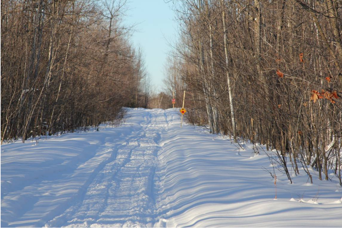
Figure 26 View of first stop ahead - stop sign combination - placement is 275 feet (warning sign to stop sign) on a high speed section of trail.
